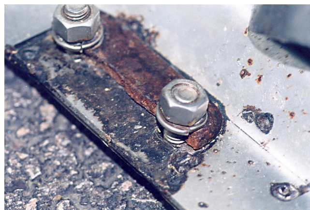
Fig. 2 — Close-up of the remains of a bracket attached to a baffle after failure.
