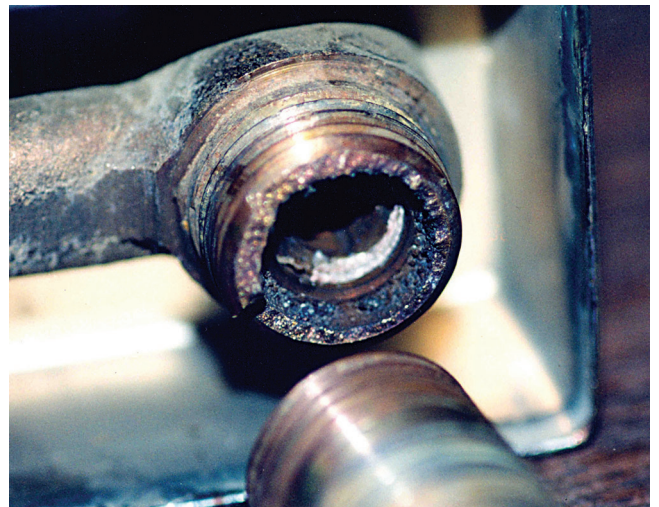
Fig. 2 — Fracture area of cast brass faucet fixture.
